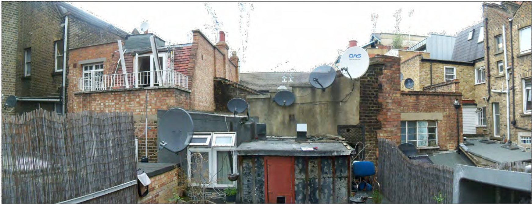
Existing Rear Photos
