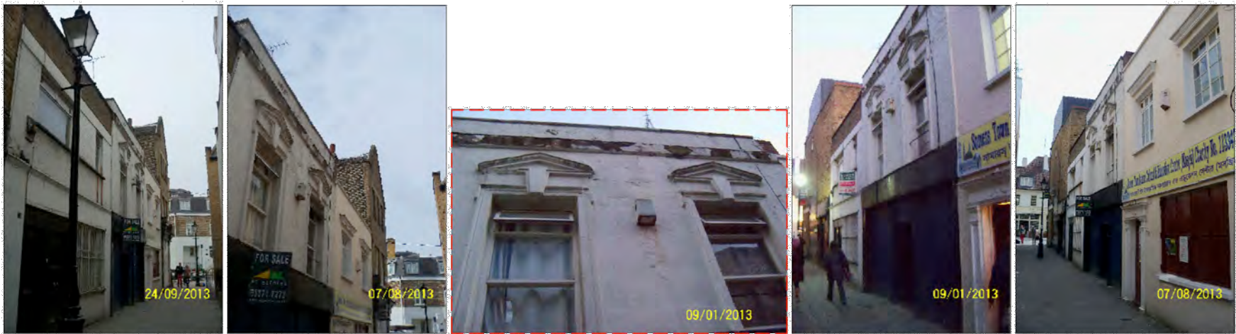
Existing Front Photos
