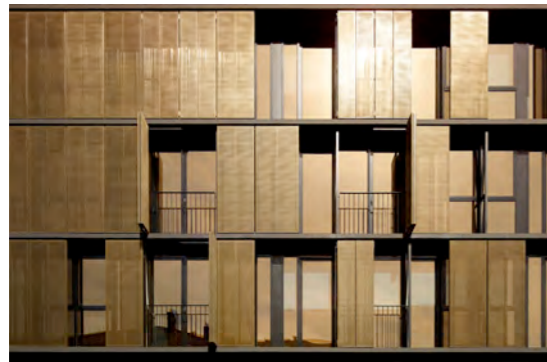
Luna Apartments: Melbourne Example of glazed building with bronze transparent mesh screen
