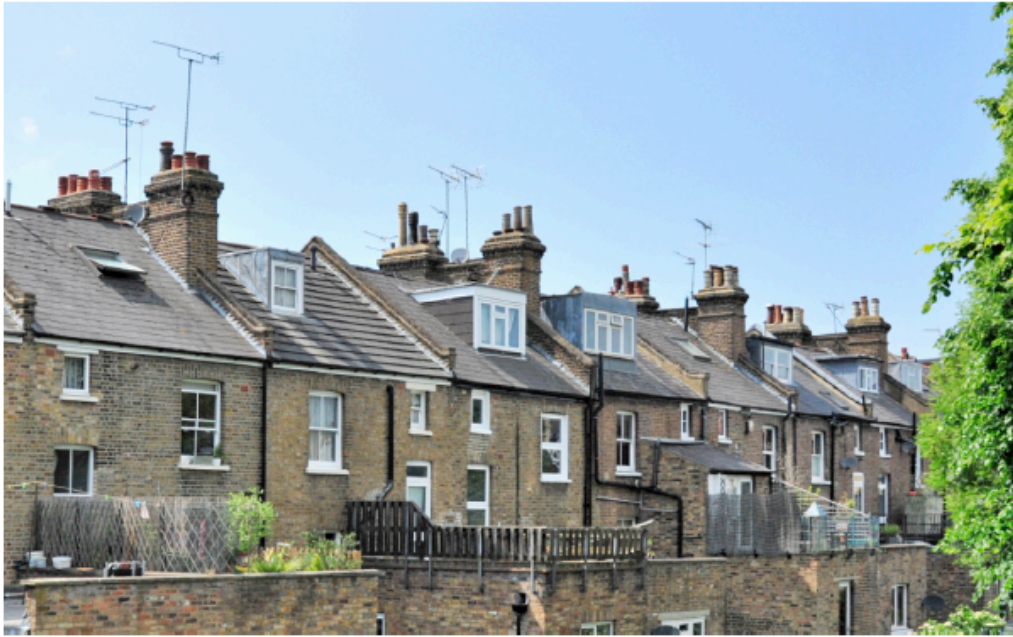
6 Dormers to rear of Roderick Road
