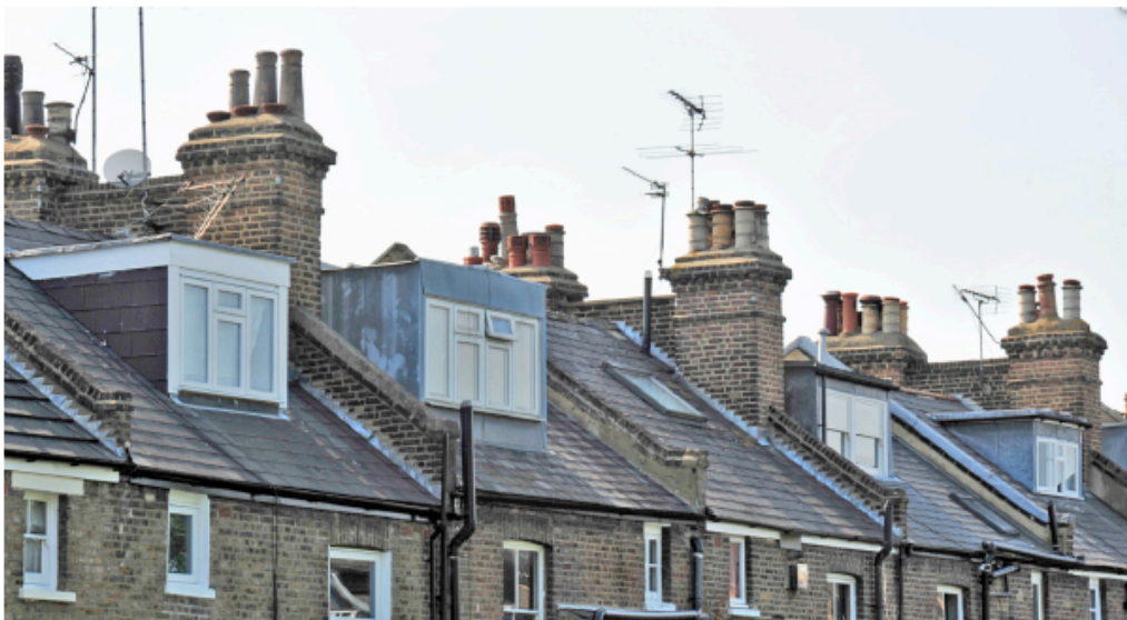
7 Enlargement of above, showing majority of metal clad dormers and rather suburban looking slate tiled dormer in foreground
