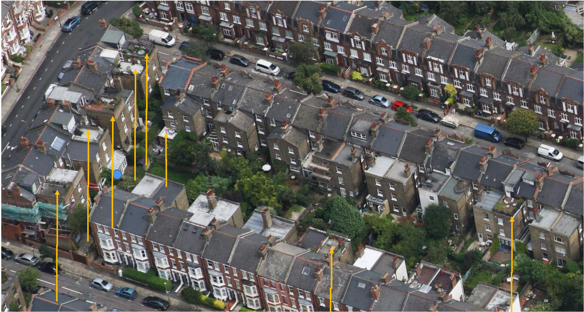
Samples of other roof terraces in the area
