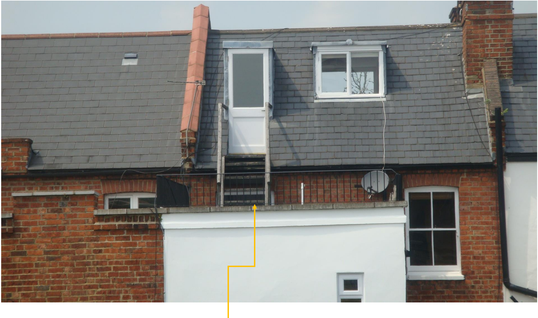
Samples of other roof terraces in the area
