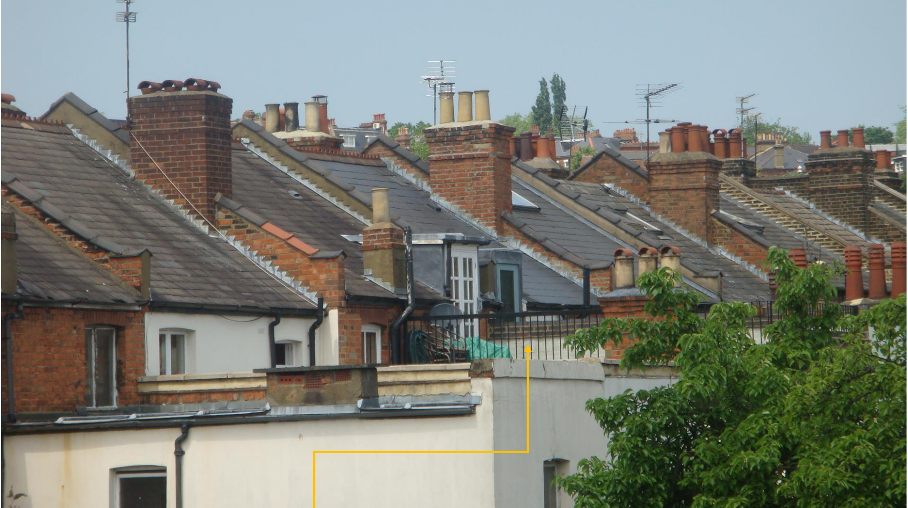
Samples of other roof terraces in the area
