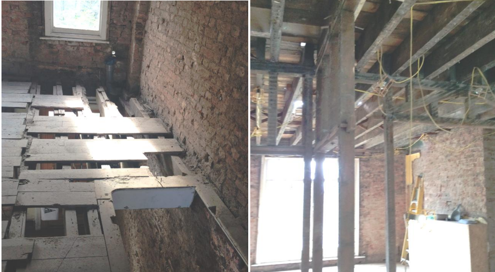
EXISTING STRUCTURAL CONDITION OF THE PROPERTY
