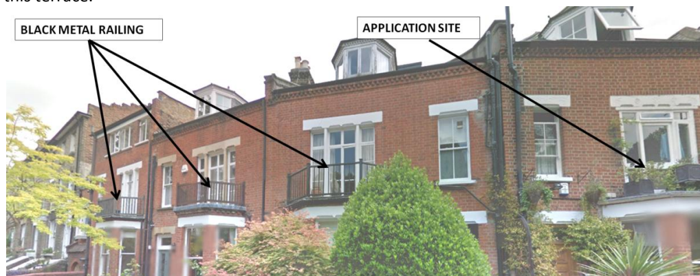
EXISTING TERRACE WITH BLACK METAL RAILINGS
