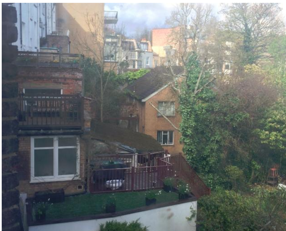
FLAT ROOF REAR EXTENSIONS AND TERRACES IN THE NEIGHBOURING PROPERTIES
