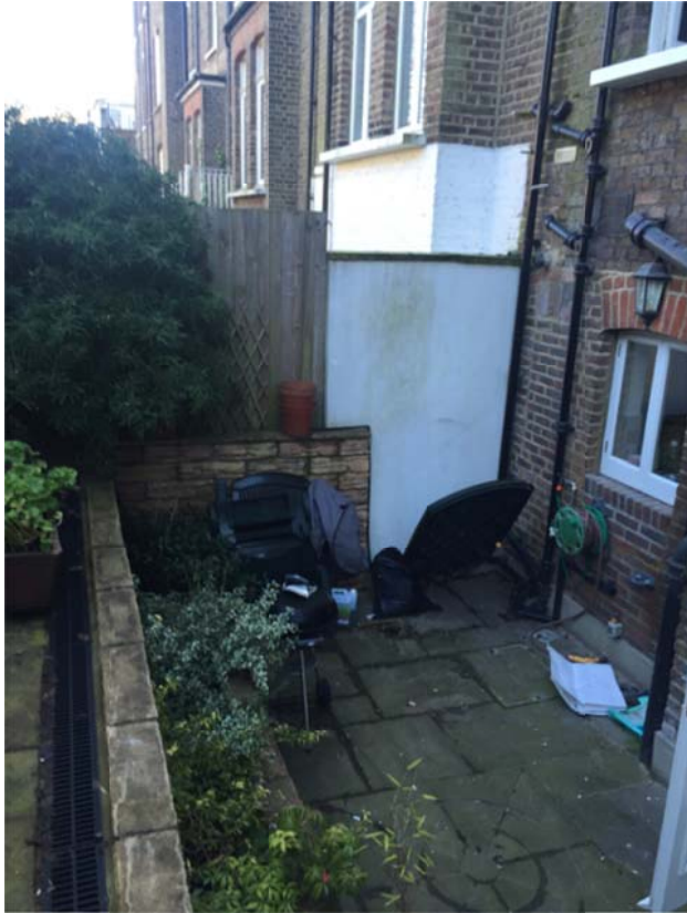
Patio and boundary wall to no. 16
