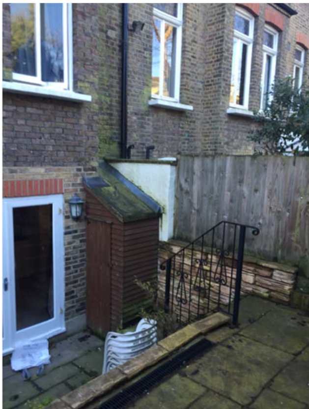
Patio and boundary wall to no. 20
