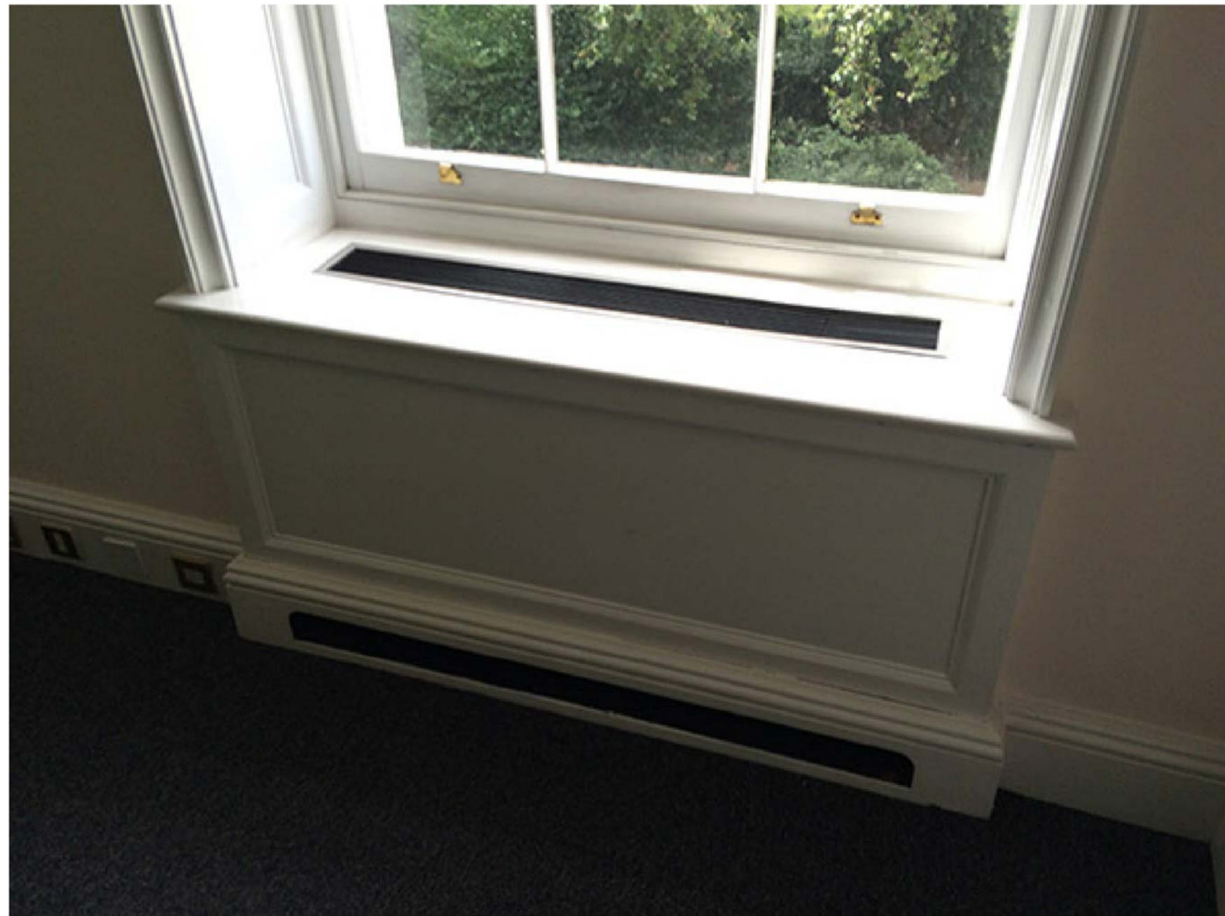
03 - Photo of existing timber boxes built into window reveal
