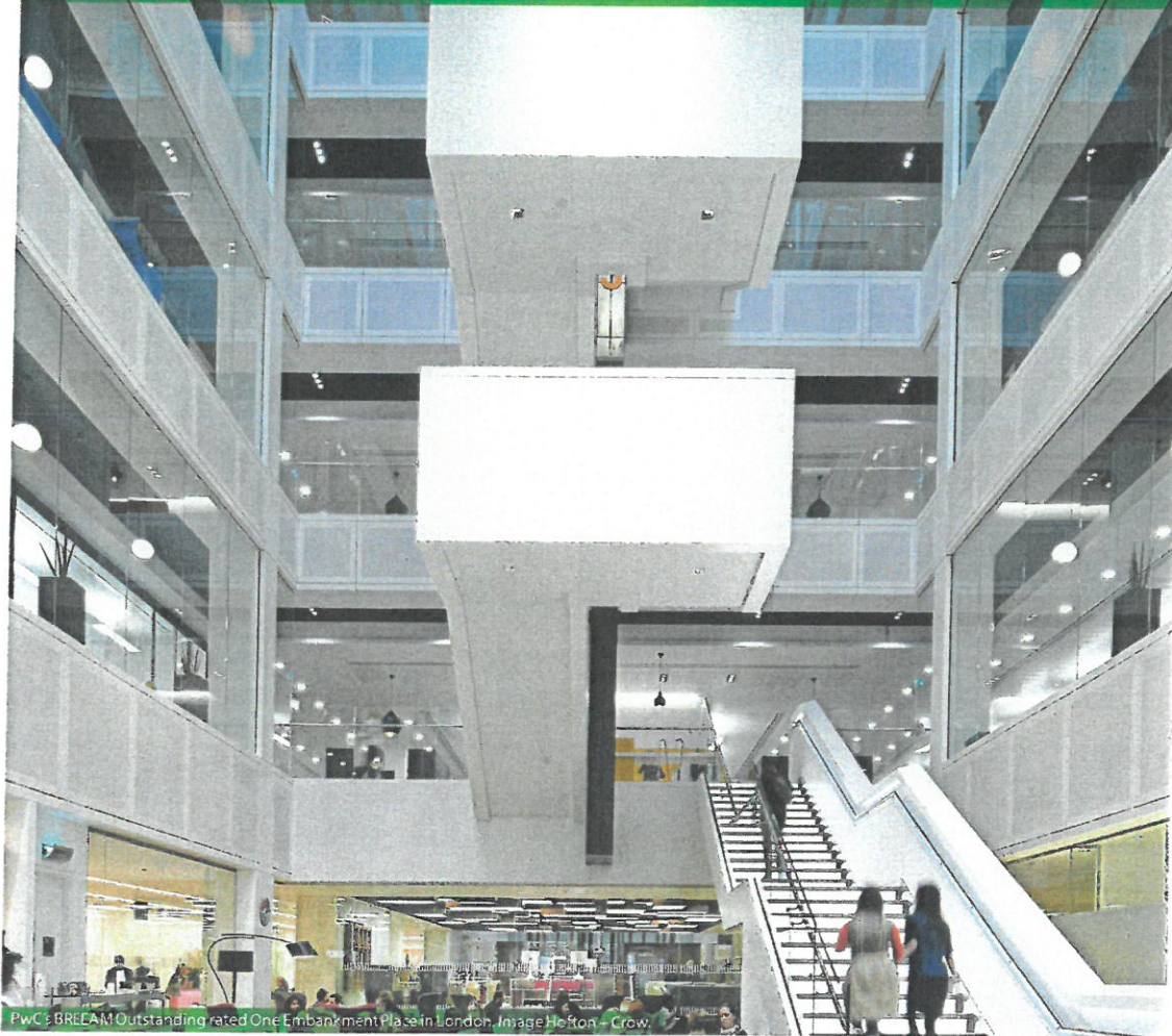
PwC's BREEAM Outstanding rated One Embankment Place in London. Image Horton - Crow.
