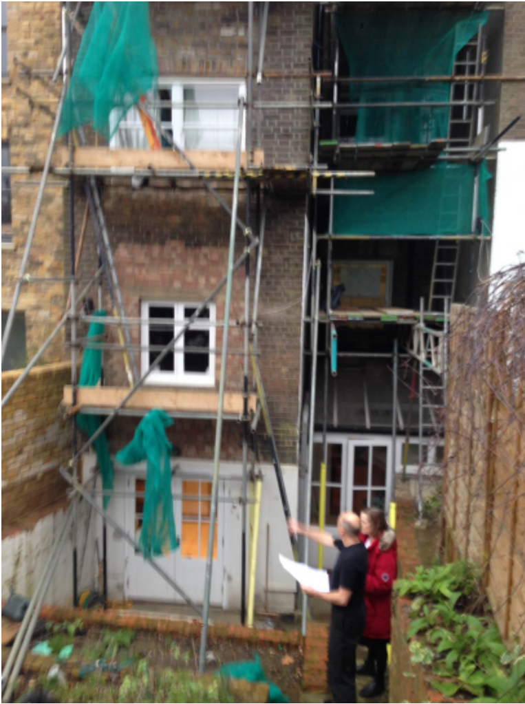
1. View towards rear elevation
