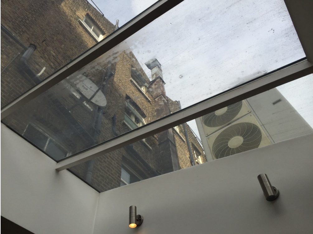
View of rear elevation to existing air conditioning units at 35 Theobald's Road
