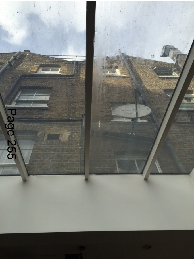
View of rear elevation via ground floor roof lights
