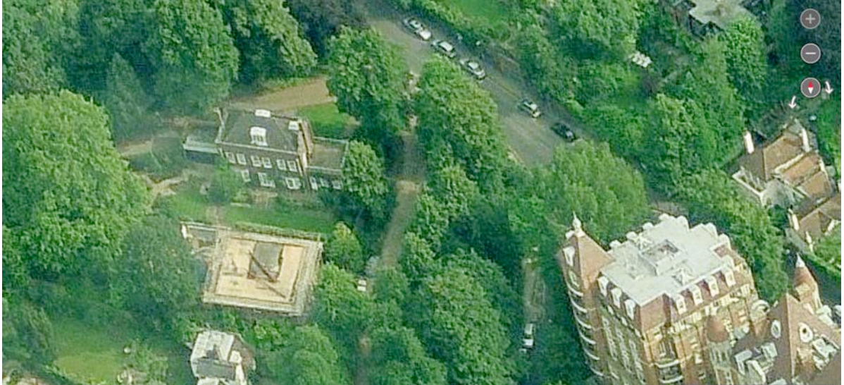
Aerial view looking east, with No. 115 Frognal on the left, and the former, listed Frognal Grove on the right.
