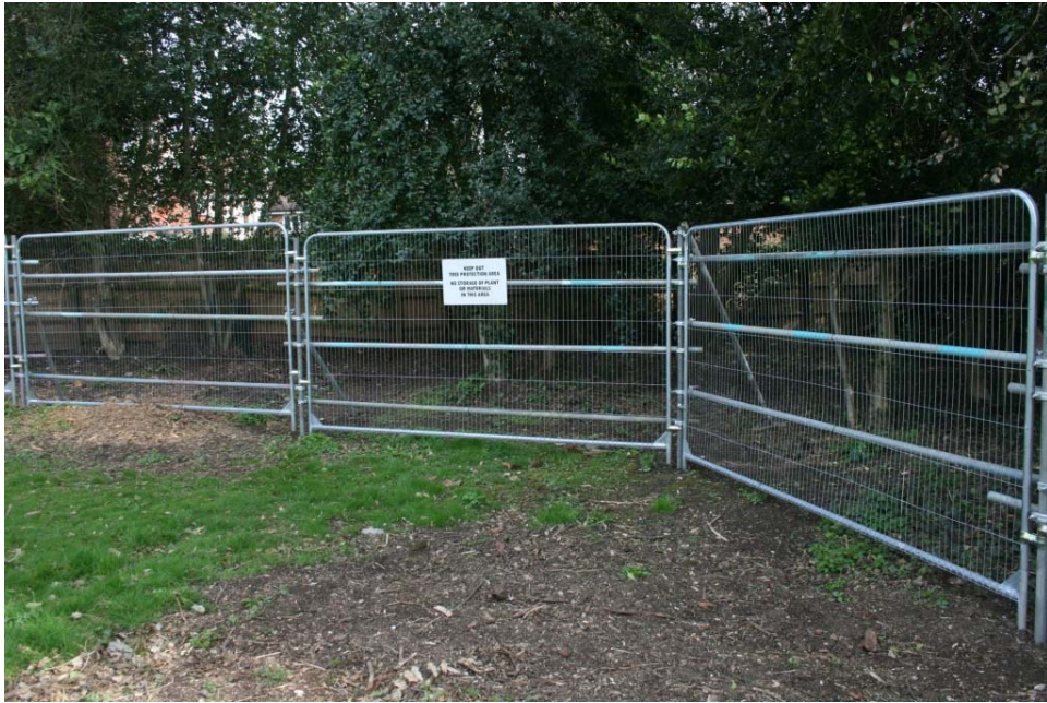
Photograph 1: showing example of TPF erected to the correct specification
