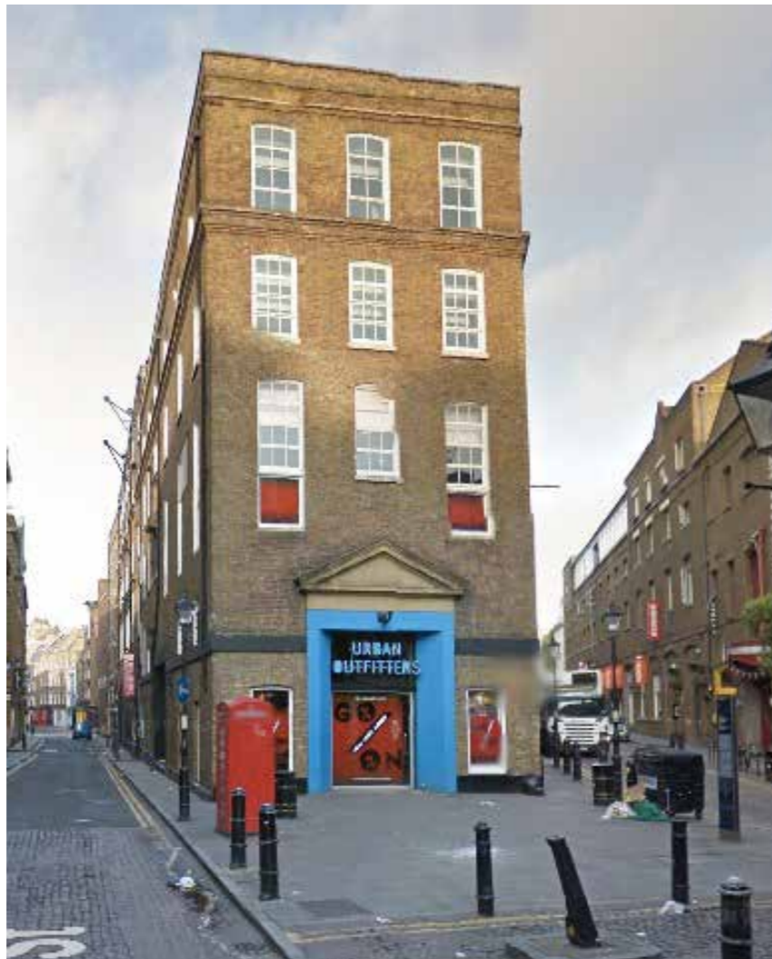
17. Front elevation of the Seven Dials Warehouse facing onto Five Dials Square 2016 (DIA)
