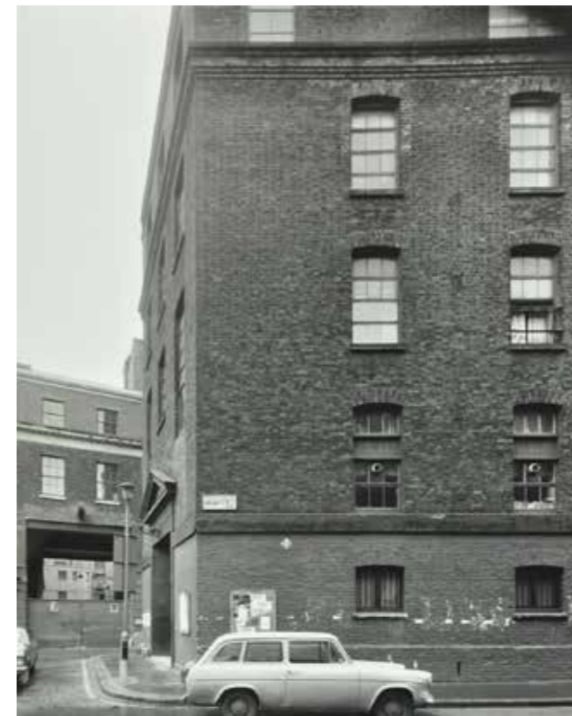
11b. Photograph of the Earham Street elevation of the Seven Dials Warehouse, 1975 (Collage)
