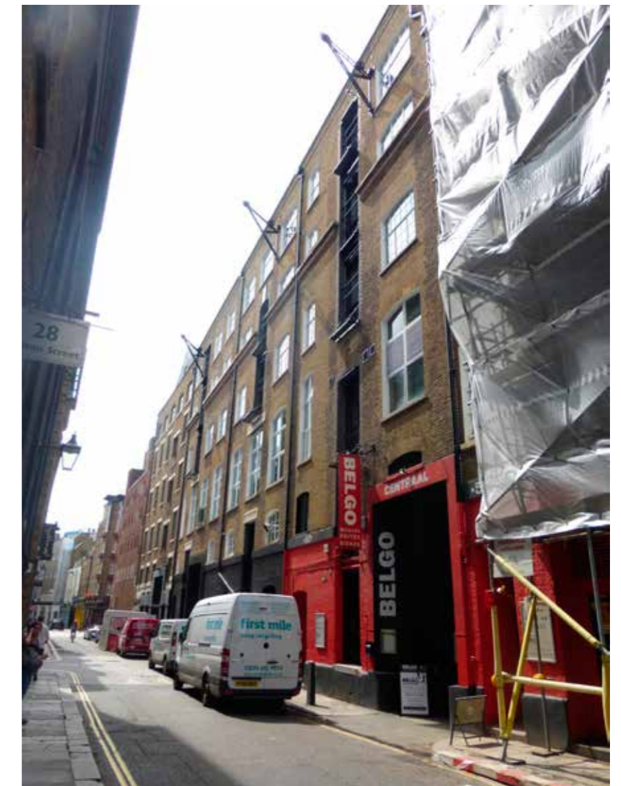
18. Side elevation of the Seven Dials Warehouse facing onto Shelton Street, 2016 (DIA)
