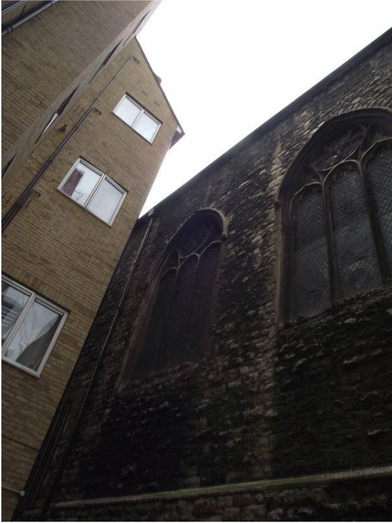
Flats and upper elevation of church
