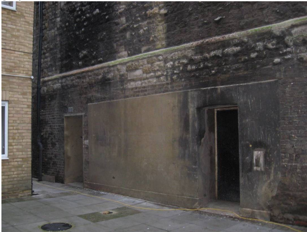
Basement vault fire escapes
