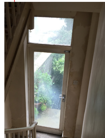
First floor landing rear window showing existing original single glazed sash window in poor condition PROPOSAL- replace window to match original
