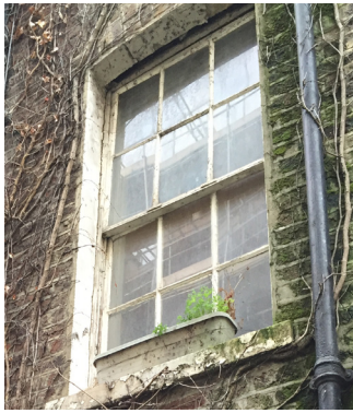
Second floor existing rear window not original- replaced in the 1970's with the refurbishment of the roof PROPOSAL- replace window to match original
