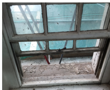
Ground floor rear window showing existing original single glazed sash window in poor condition PROPOSAL- replace window to match original
