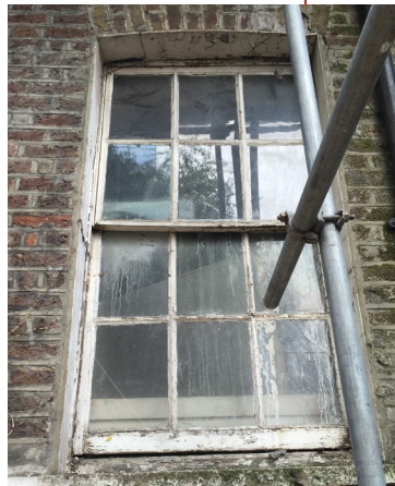
First floor existing original rear window showing single glazed sash window in poor condition PROPOSAL- replace window to match original
