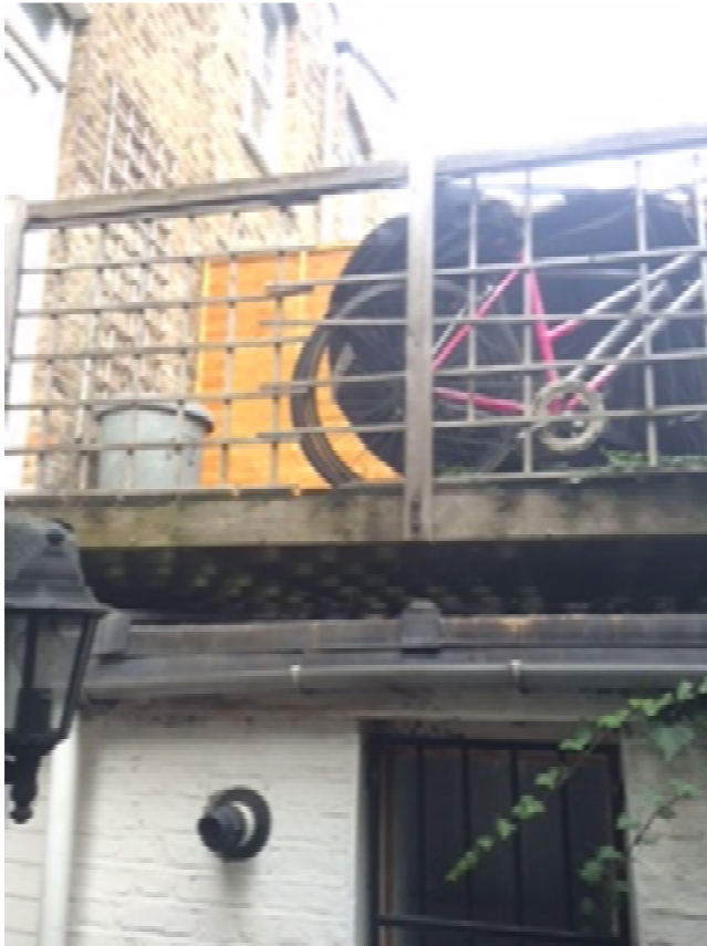
Existing terrace at ground floor flat
