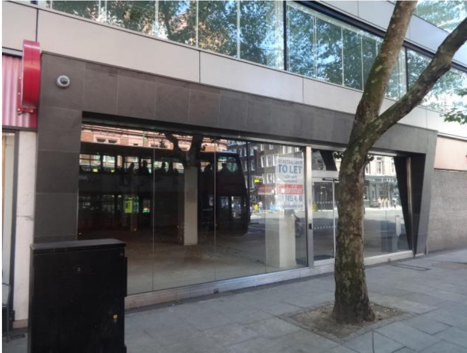
Photo 1 – Front view of unit 133 Clerkenwell Road – application site. Slate surround to be retained.
