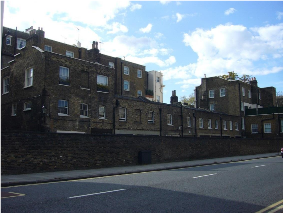
VIEW FROM ALBANY STREET
