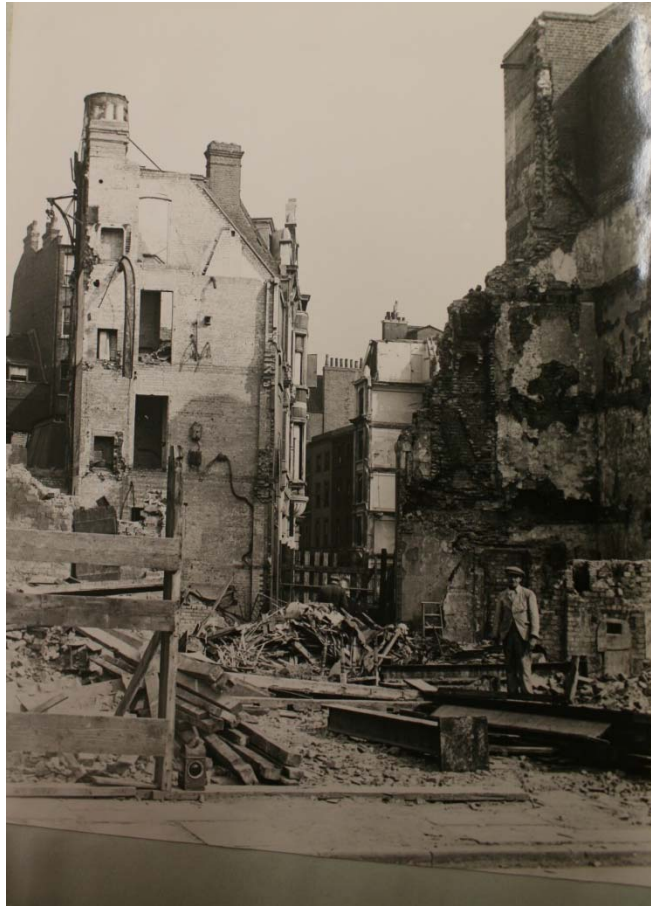
Plate 8: Bomb damage in Greys Inn Passage, looking east from Red Lion Street (Camden Local Studies and Archive LP 2681)
