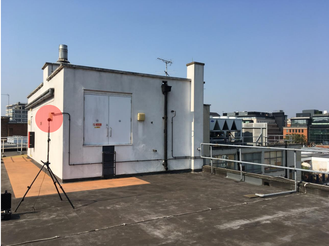
Figure 3 Photograph showing the location of measurement position L
