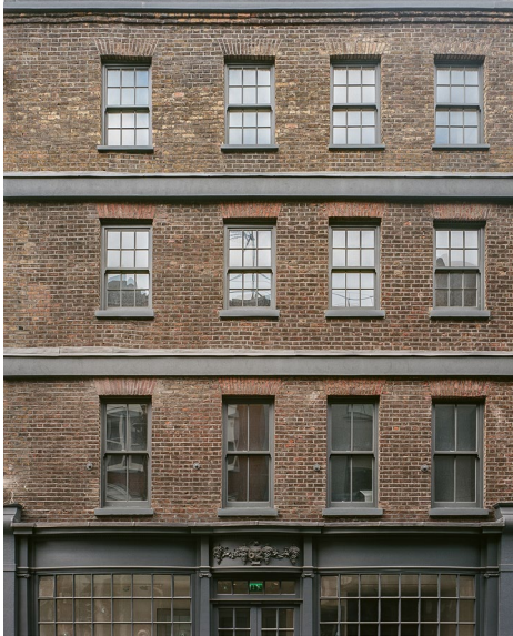
Fig 4. Grade II listed restoration and conversion to residential on Dean Street in Soho
