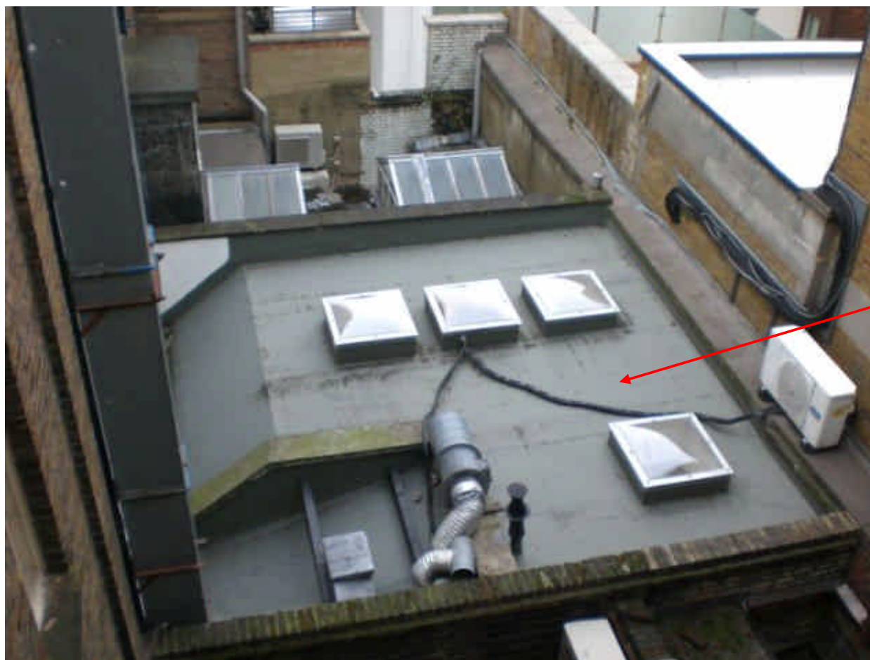
View of neighbouring roof areas
