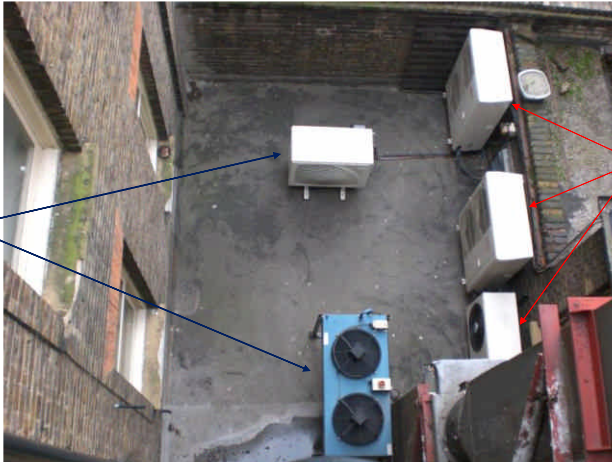
Aerial view of existing mechanical plant on flat roof
