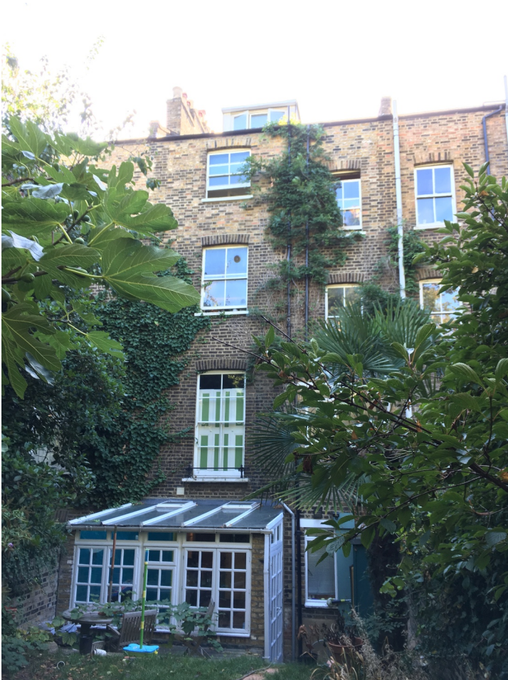
Rear of 24 South Villas. 24A occupies the ground and first floors of the property.
