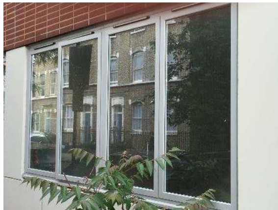
Photograph 2: Powder coated aluminium casement windows at 20a – 50 Millman Street
