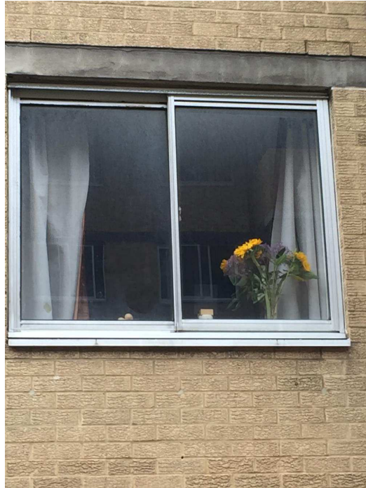
Photograph 1: Existing aluminium horizontal sliding sash window at Jeygrove Court
