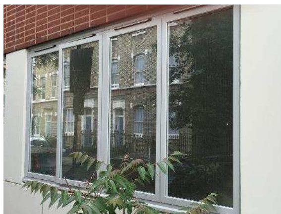
Photograph 2: Powder coated aluminium casement windows at 20a – 50 Millman Street
