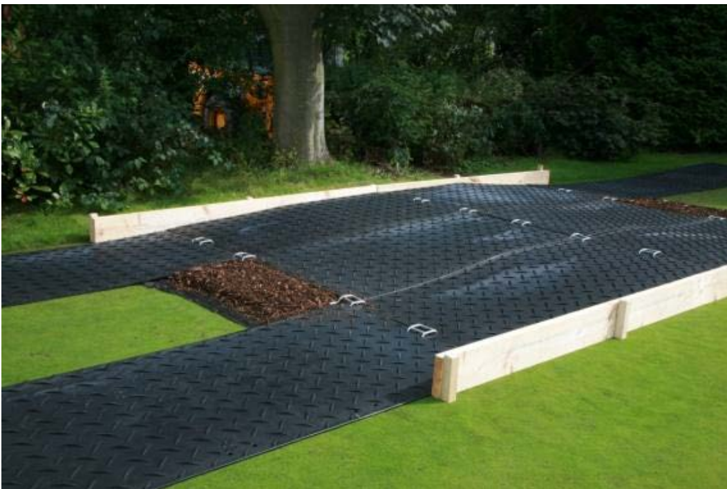
Ground-Guards, installed using a geotextile membrane, ground panels, 150mm deep woodchip and ground panels on top and held in place with edge rails. Please refer to www.ground-guards.co.uk/ for more details.
