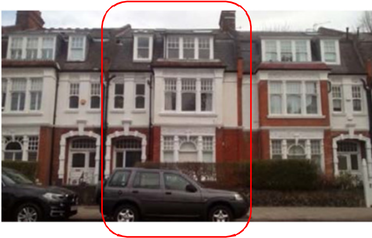
View of street elevation with application site shown in red
