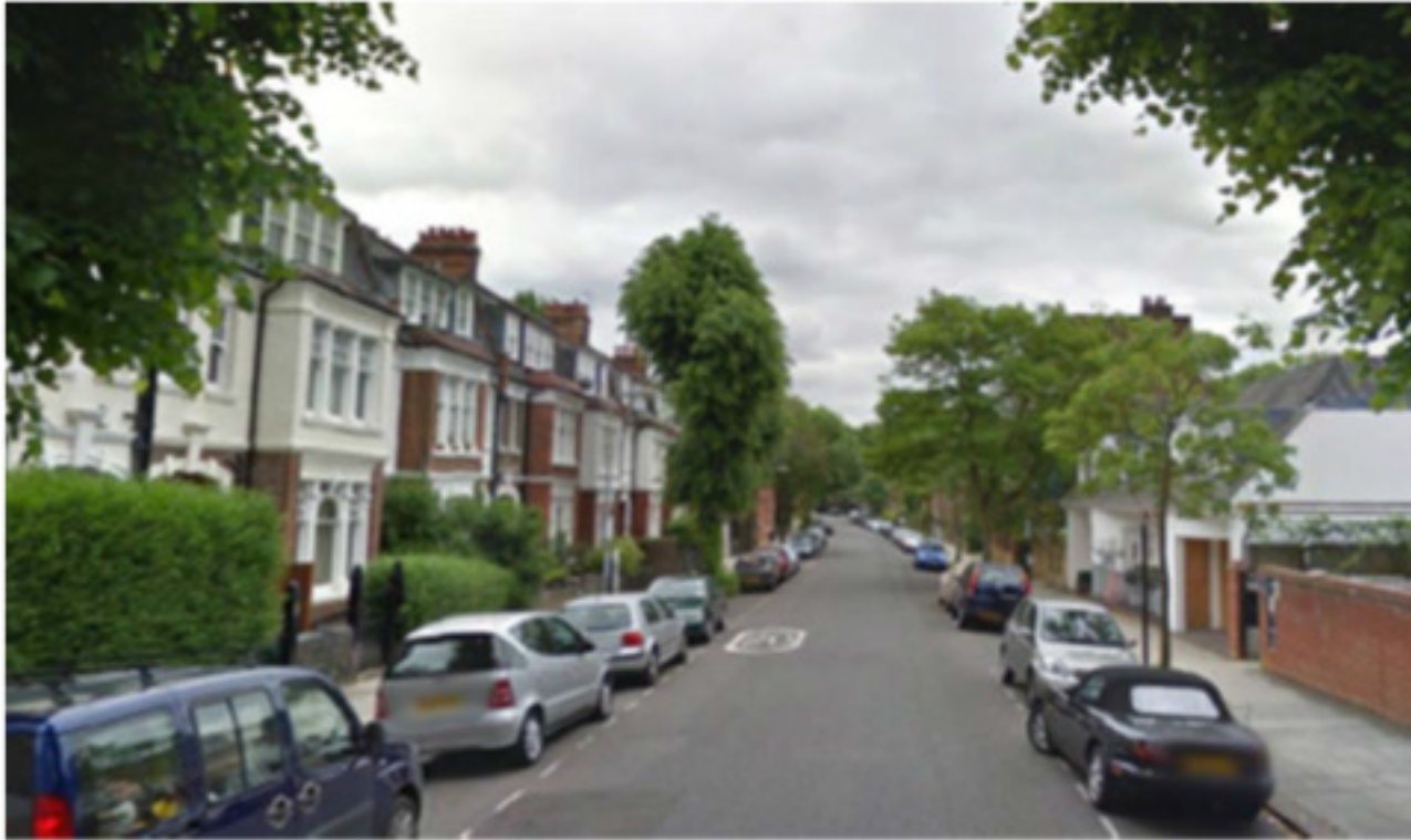
View of Glenilla Road looking south west with application on the left
