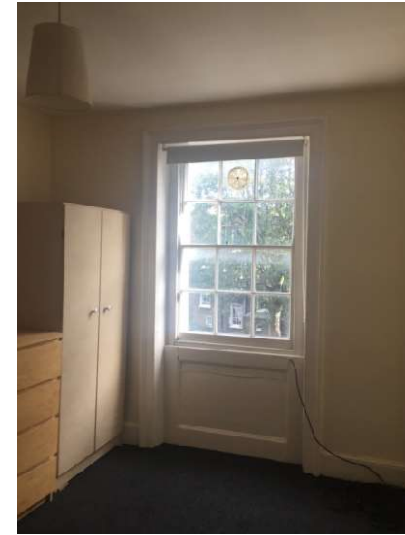
Plate 14. Original window, modern bottom sash
