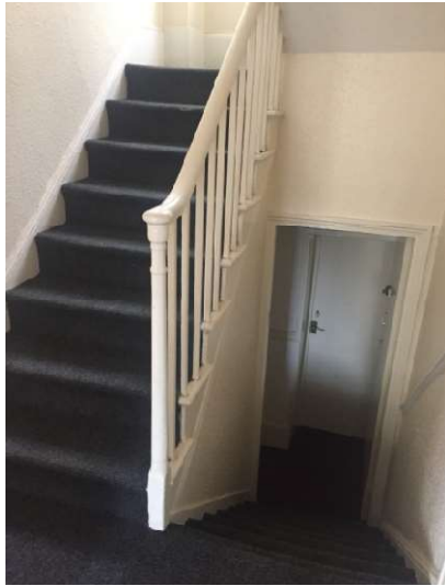
Plate 12. Ground to first floor flight
