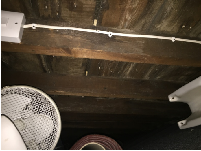
Plate 16. Modern roof timbers and close boarding
