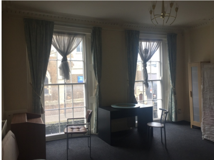
Plate 8. Front room, original cornice, skirting and top sashes
