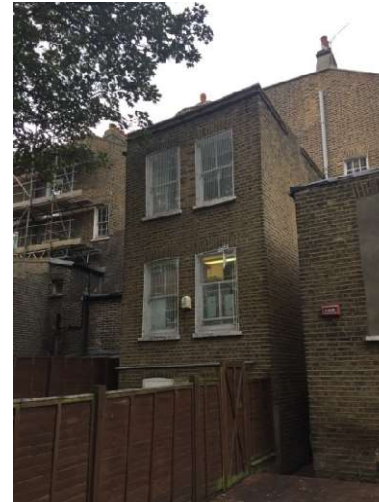
Plate 18. Three storey extension to No.22
