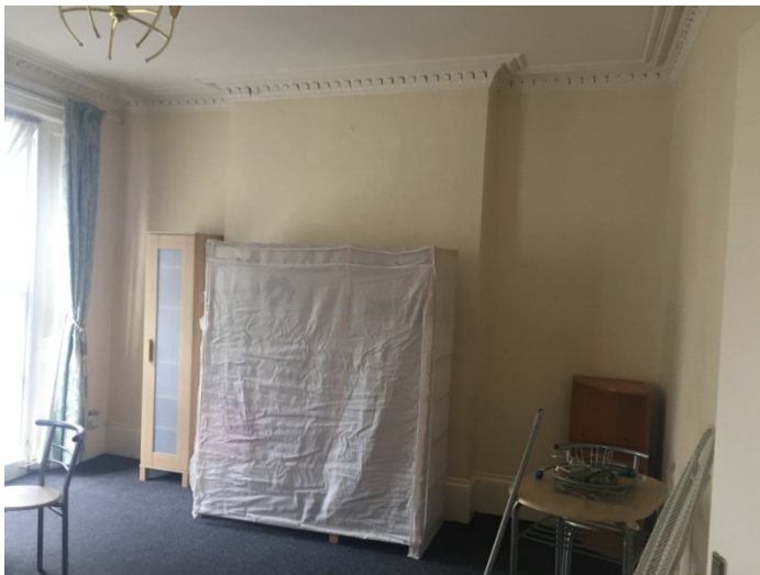
Plate 9. Original chimneybreast. No original fireplace survives
