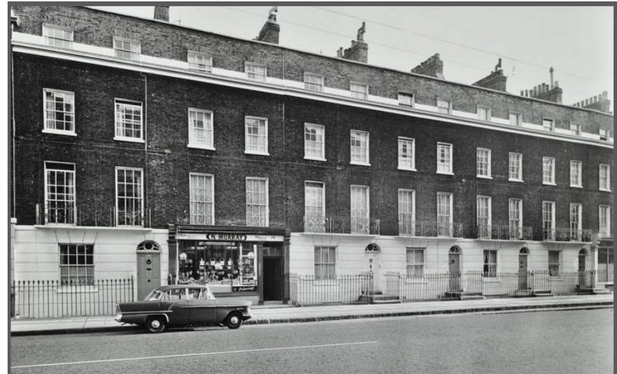
Plate A. Nos.50-60 Camden Road, dated 1960 (Source: The LMA Picture Archive; Record 106626)
