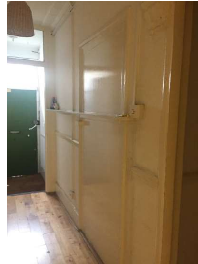
Plate 7. Original doorway, now blocked, & corbel
