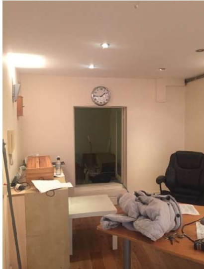
Plate 4. Original window opening
