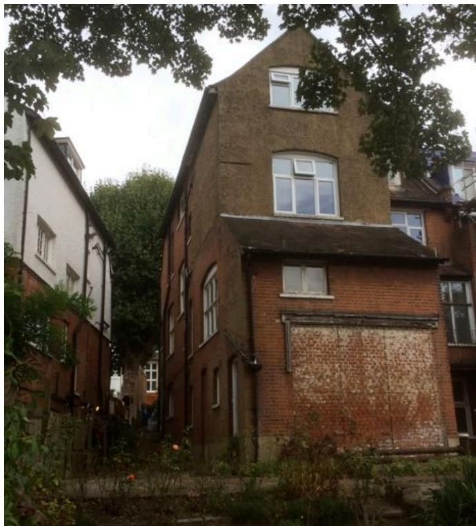
IMAGE B – Existing Rear View as seen from the garden
