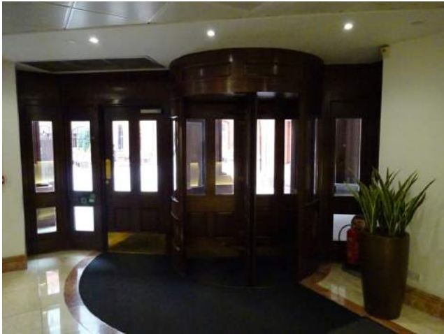
Entrance doors to be retained
