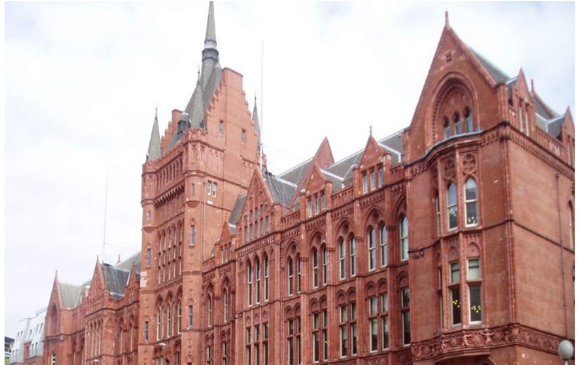
Waterhouse Square's impressive frontage onto High Holborn
