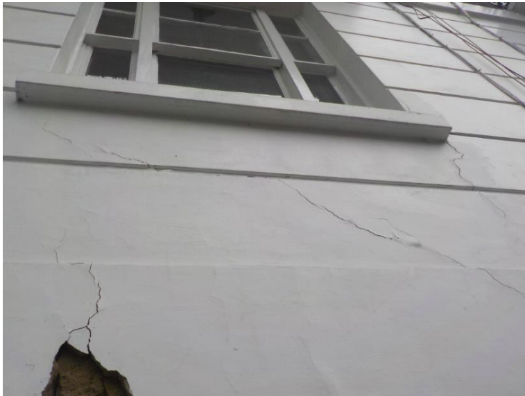
Between ground and lower ground floor window
