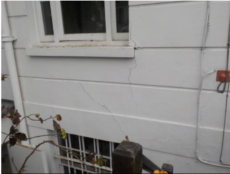
Between ground and lower ground floor window
