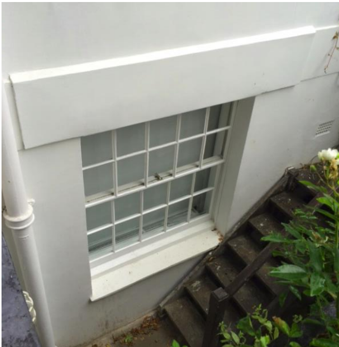
Lower ground floor window (not visible from street level)
