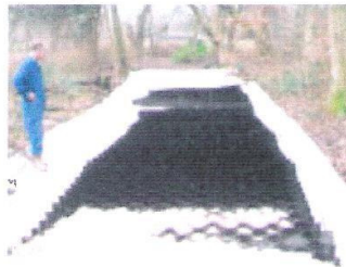
Installation of the CellWeb™ system.
