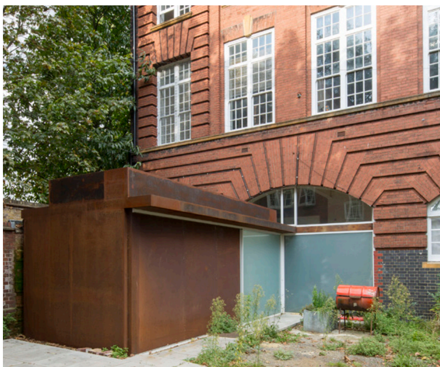
Left: Studio 3, a COR-TEN extension to the Grade II Listed Stepney Jewish Primary & Infants School London E1
