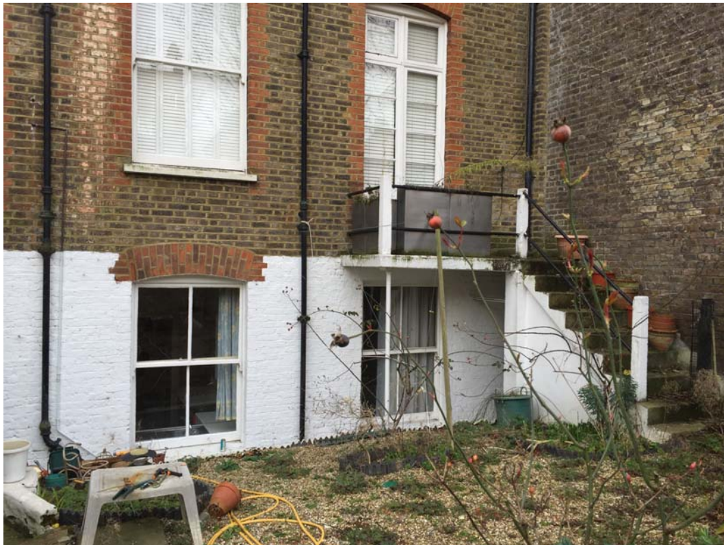
View to the rear of 134
