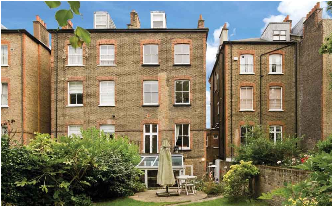
View to the rear of no.132
