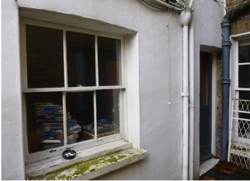
Window and side door
