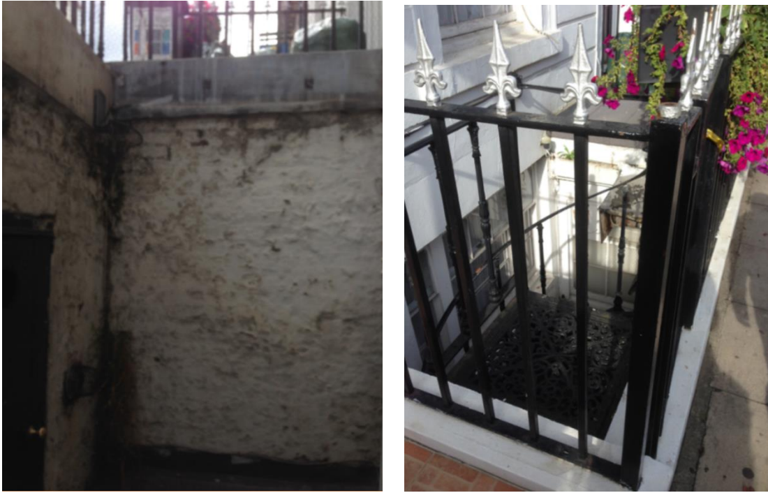
Images 6.4: Illustrating Former External Staircase and Neighbouring External Staircase
