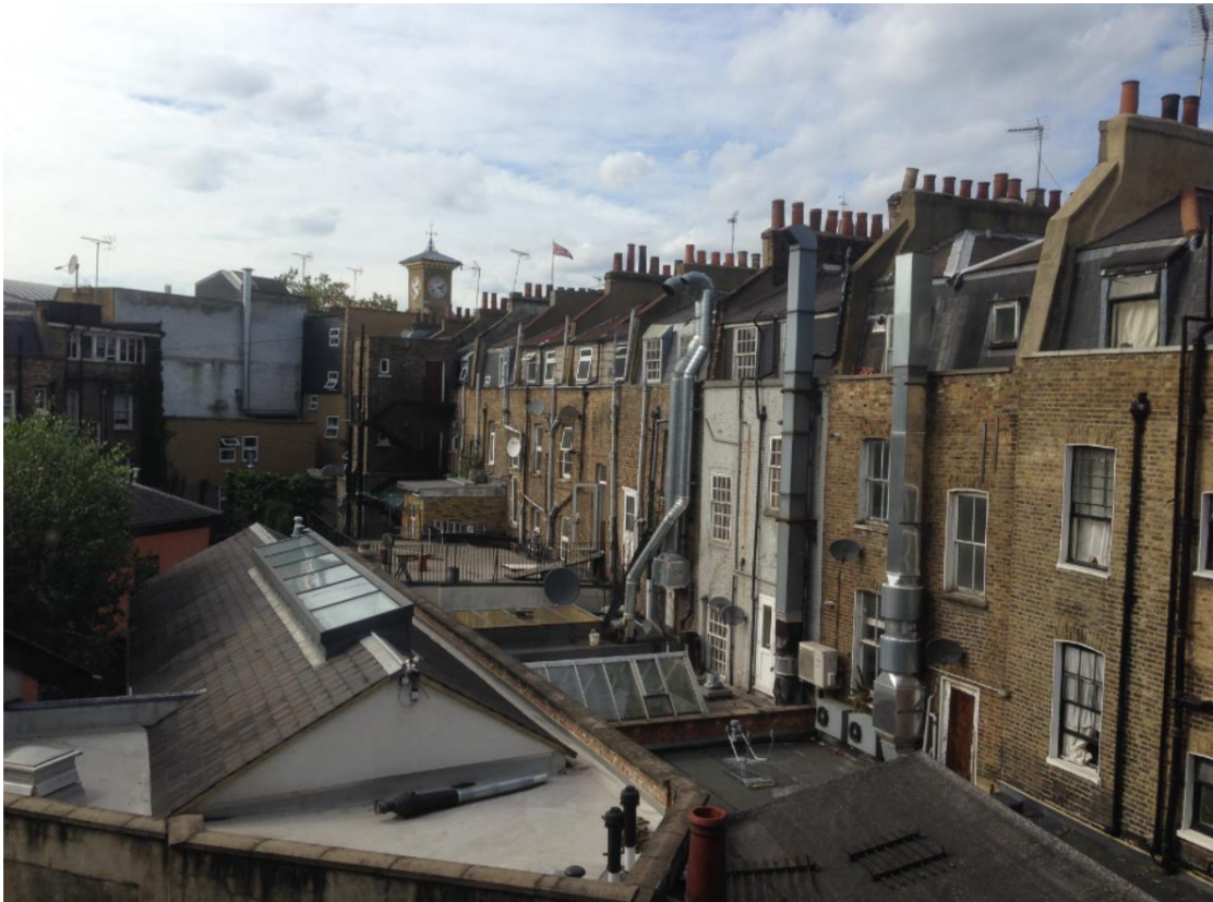
Image 6.2: Wider Setting of the Listed Building to the Rear
