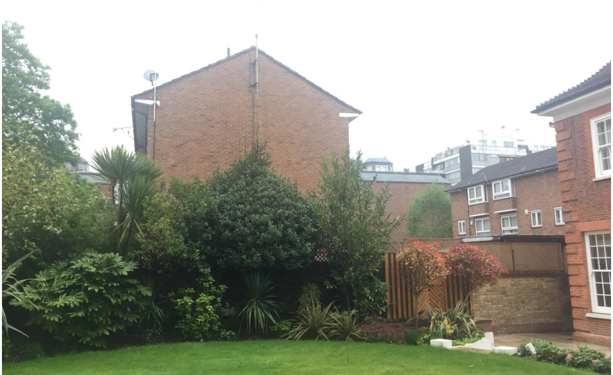
Figure 5 - The flank of the adjacent residential terrace to the south
