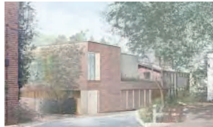
3 ADMIRAL'S WALK - SHANTON WILLIAMS ('16) - UNDER CONSTRUCTION
