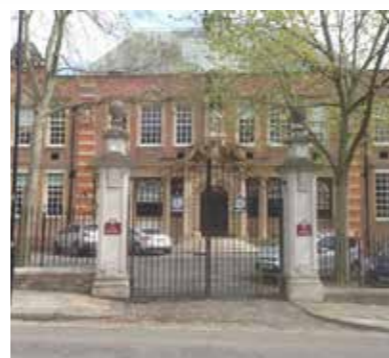
Gate 4: vehicle exit - electronically activat- ed with sensor
