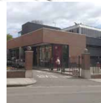
Gate 6: vehicular entry gates open from 6.30am -10.30pm. Manual operation
