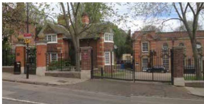
Gate 1: pedestrian entry to lodge -locked.
