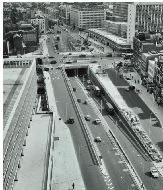
Figure 3.11: Rooftop view looking east toward the completed Euston Road underpass in 1966 (Source: Collage, City of London)
