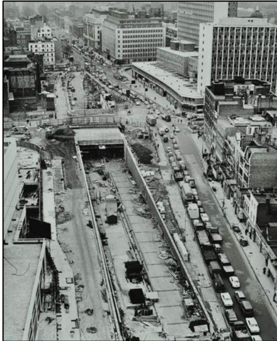
Figure 3.10: Rooftop view looking east toward the construction site of the Euston Road underpass in 1966 (Source: Collage, City of London)
