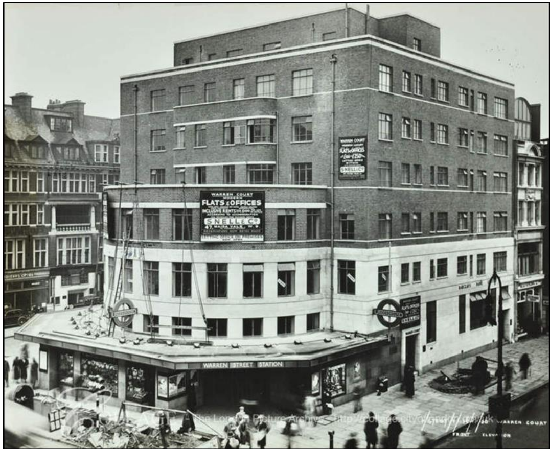
Figure 3.7: View of Warren Street Station in 1936 (Source: Collage, City of London)
