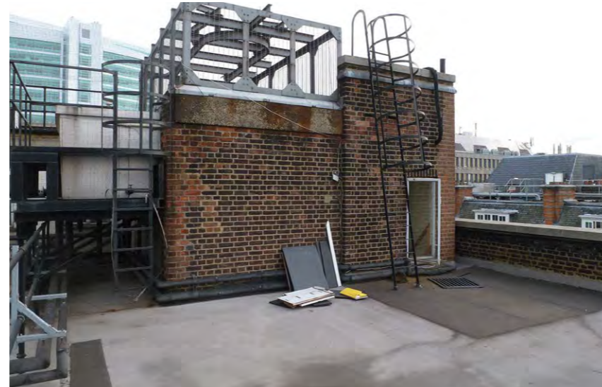
View of ladder access to roof level.
