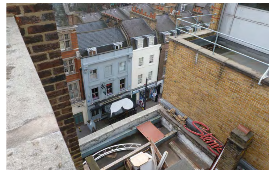
Roofscape of the adjoining building
