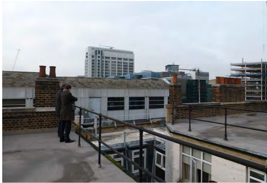
View on the rooftop to the West
