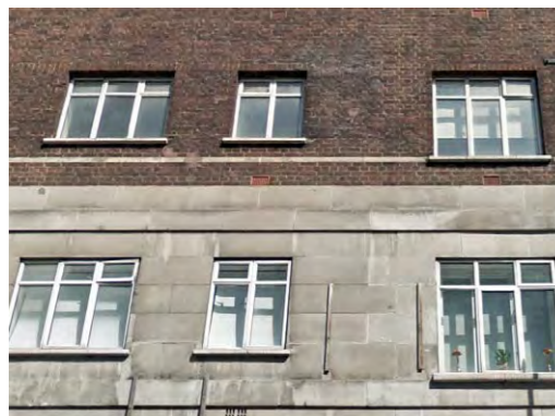
Windows - south elevation
