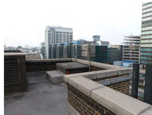
Existing roof looking west
