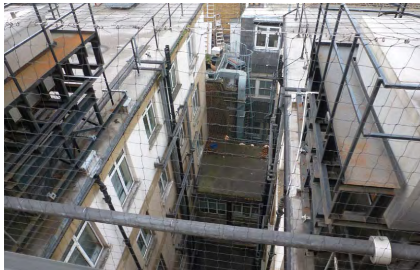
View of adjoining residential windows taken from upper floor level
