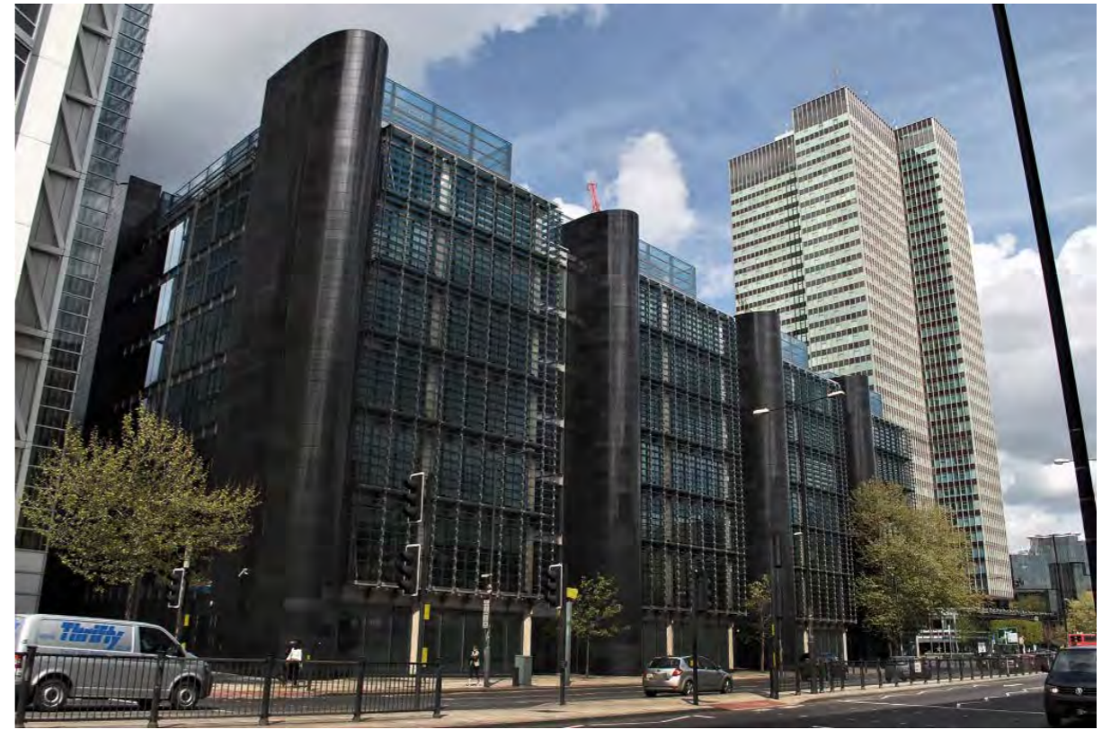
Triton Square - View of southern boundary of Regents Place from Euston Road
