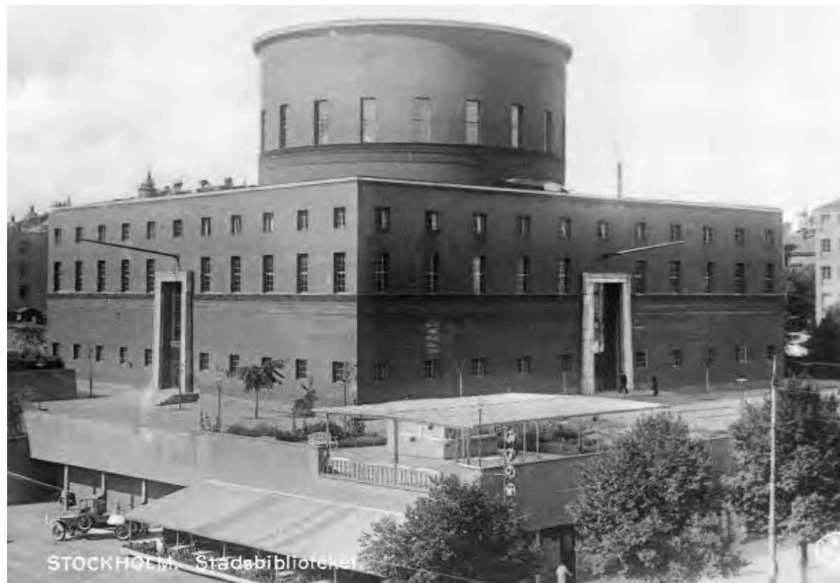
Stockholm Public Library - Gunnar Asplund, 1928, visited by Holden prior to designing Warren Street Station.
