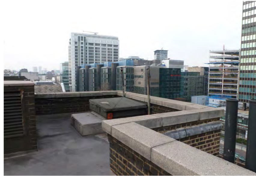
View of existing lift over run
