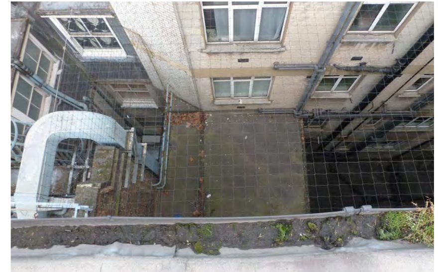
View down into the lightwell
