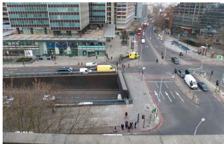
View into Euston Road underpass taken from the rooftop of the application site.
