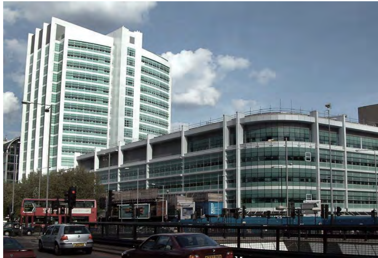
University College Hospital - (adjacent to the site) - View of north-west corner from Euston Tower.
