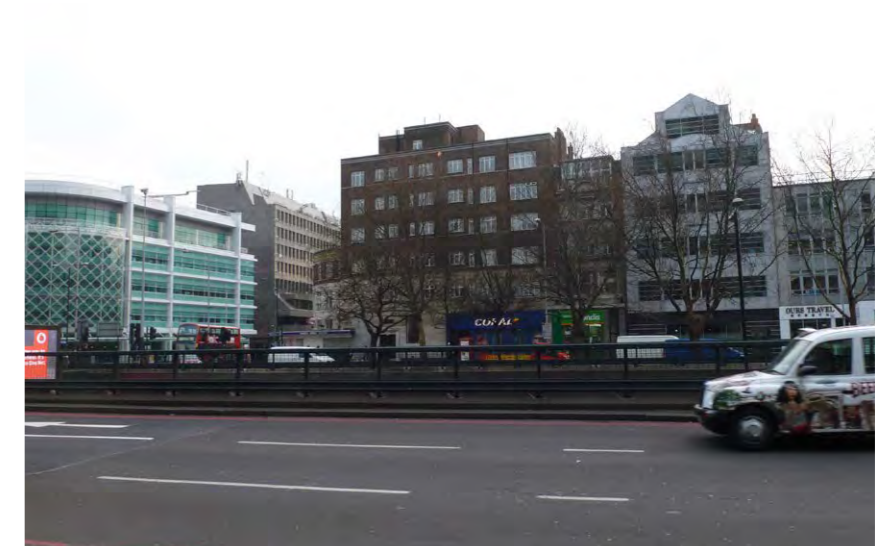
View of the site taken from the north side of Euston Road.
