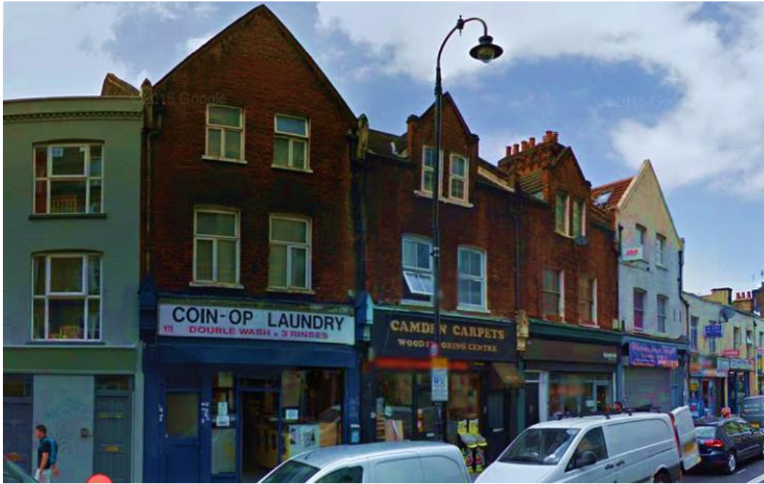
Existing front elevation of 111 Kentish Town Road
