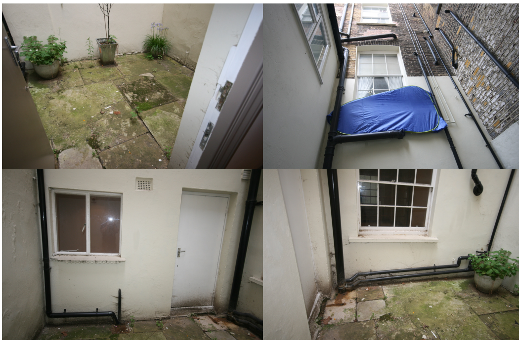
Left – Images of Rear Courtyard.
