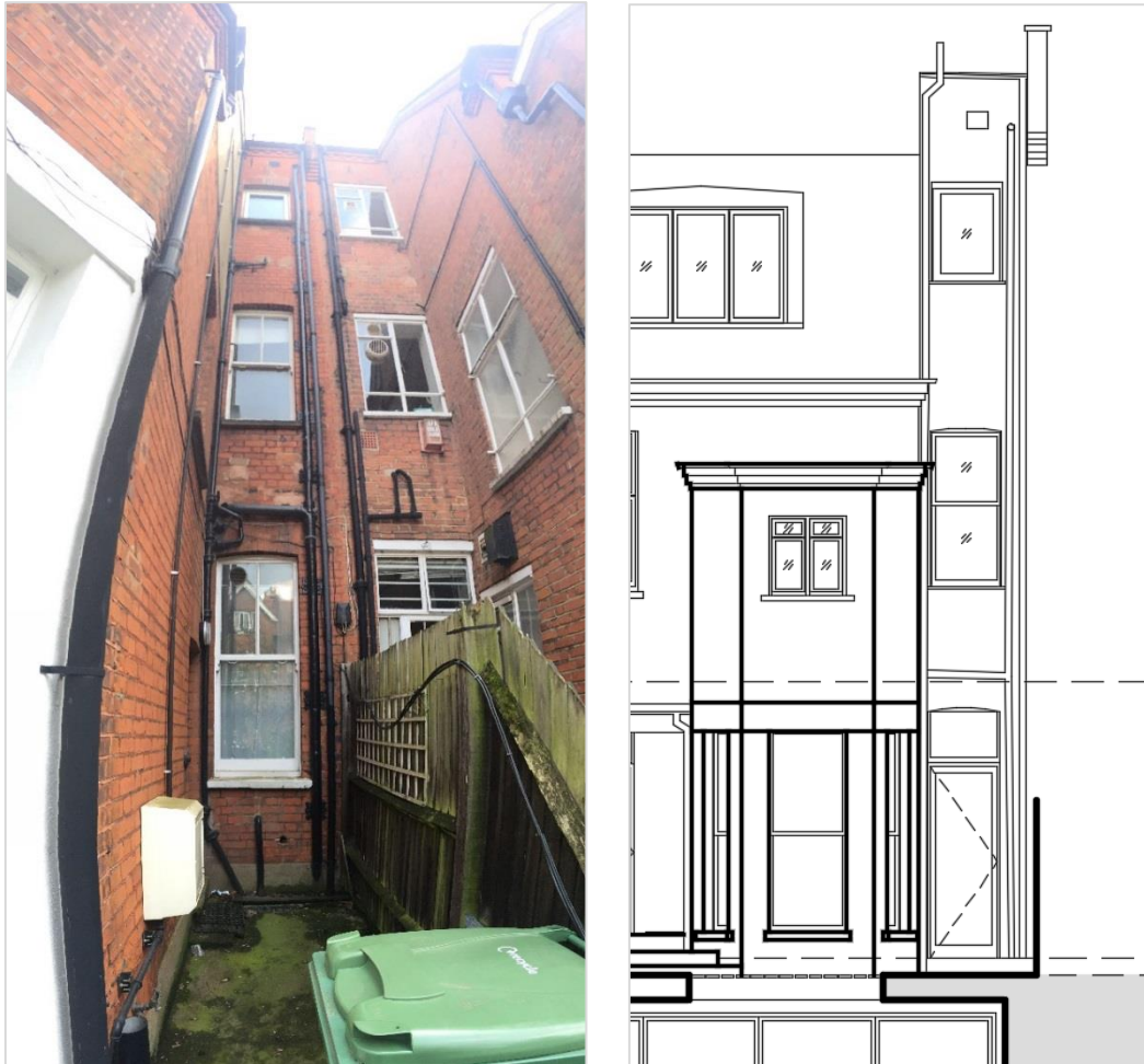
Image 8 _ Existing window to be lowered to form a new side entrance
