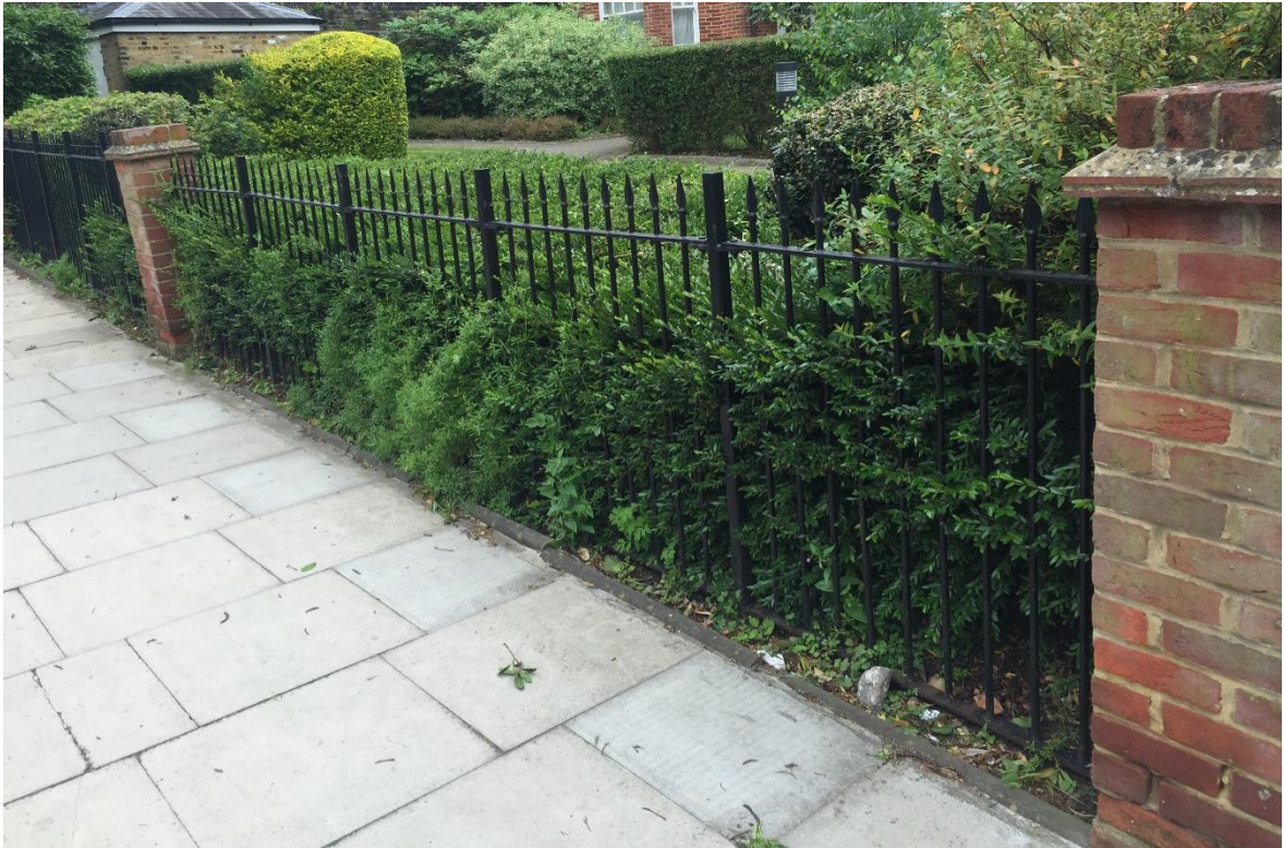
Image 7 _ Existing railings at Windsor Court
