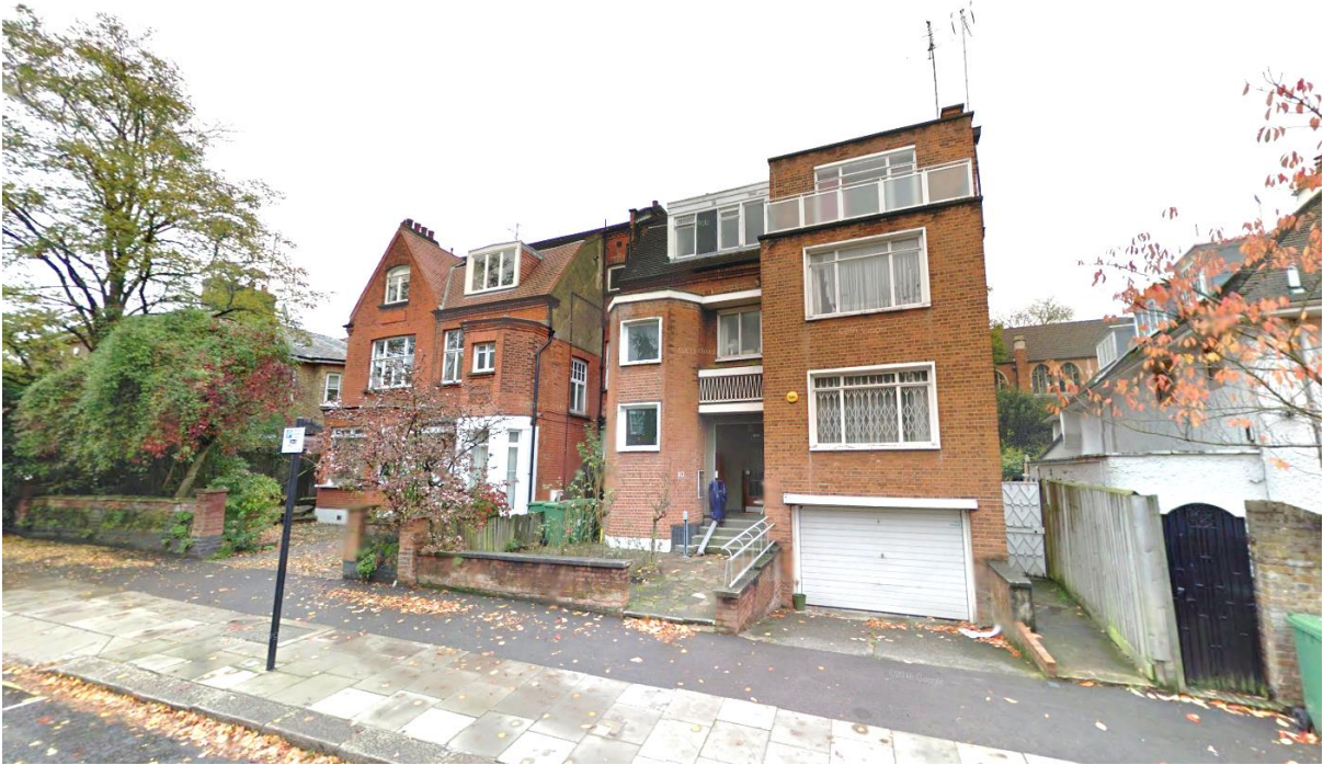
Image 1 _ the modern alterations to no.14 Platt's Lane (semi-detached)
