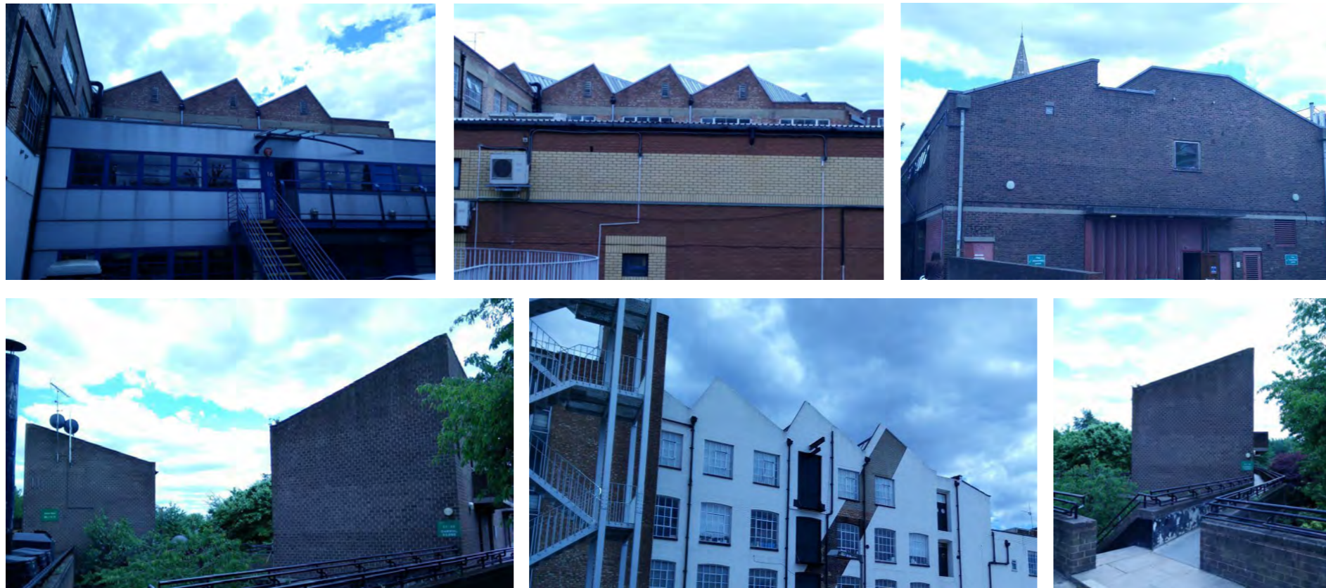
Pitched Roof Forms in the Local Area
