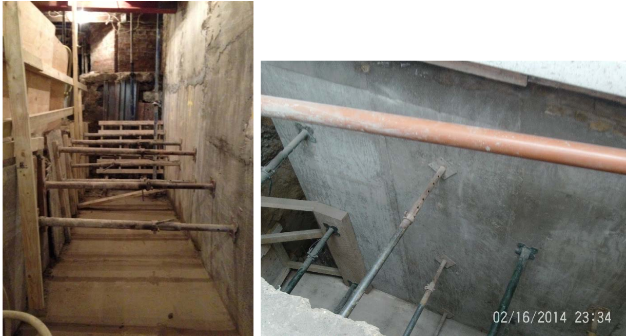
Figure 5 Examples of completed walls and back propping to central soil mass
