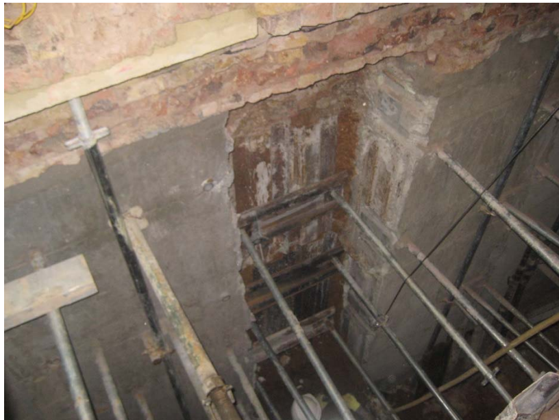
Figure 6 Example of trench sheet back propping
