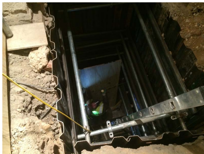
Figure 3 Propping examples
