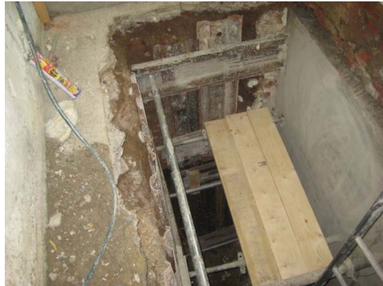
Figure 3 Propping examples
