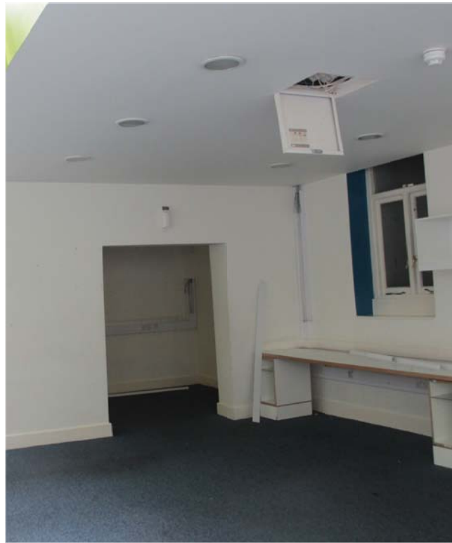
Photo 1 BASEMENT: DOUBLE DOORS to BE FITTED within EXISTING OPENING
