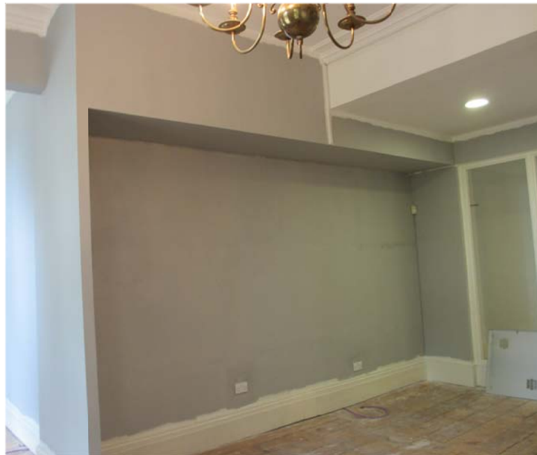
Photo 5 FIRST FLOOR: NON-ORIGINAL PARTITION to BE REMOVED; U/S of BULKHEAD RAISED
