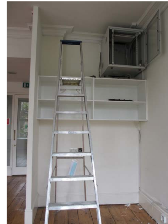
Photo 4 FIRST FLOOR: CUPBOARD DOORS w/ SIDE PANELS to BE ADDED
