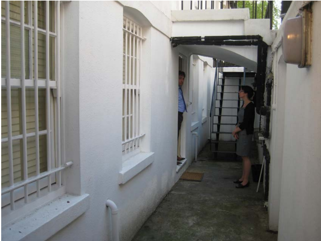
View of front lightwell
