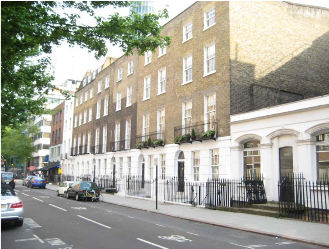
View of Fitzroy Street looking South
