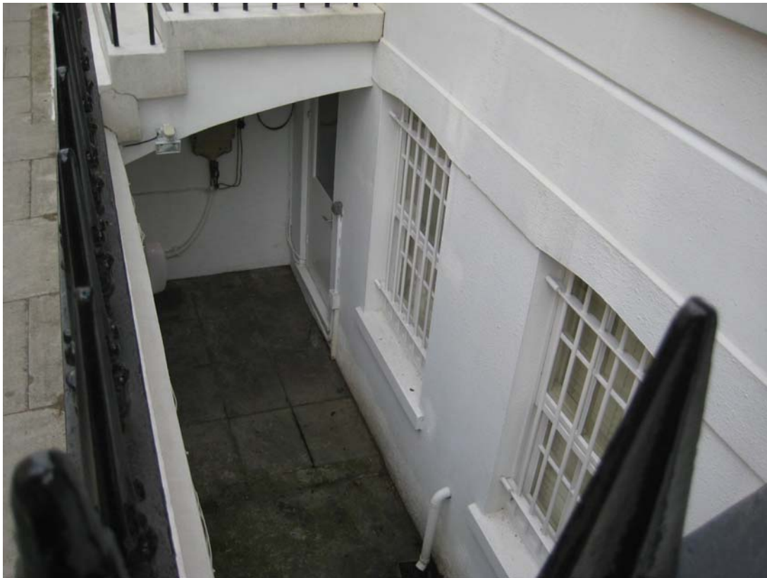
View of front lightwell (these windows are to the altered room)
