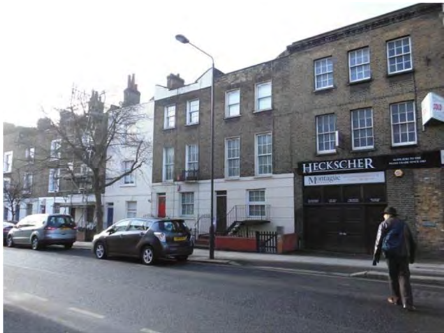
Photograph 6 - View of front of the building
