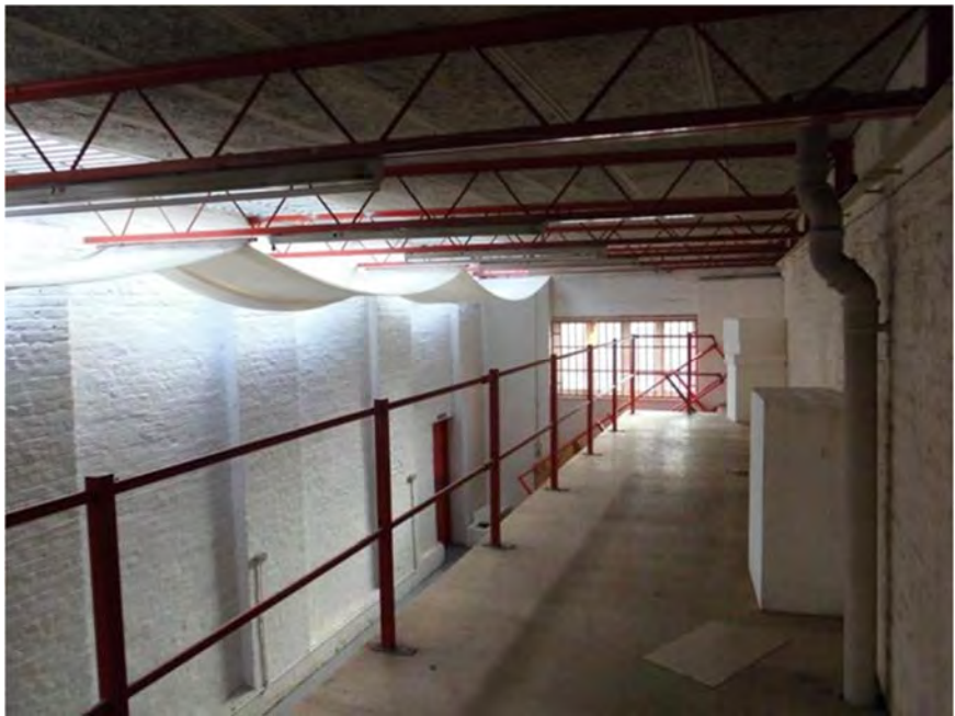
Photograph 7- Internal view of rear 'leg' of building
