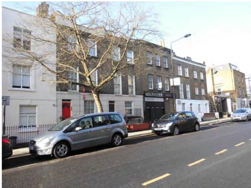
Photograph 5- View of front of the building
