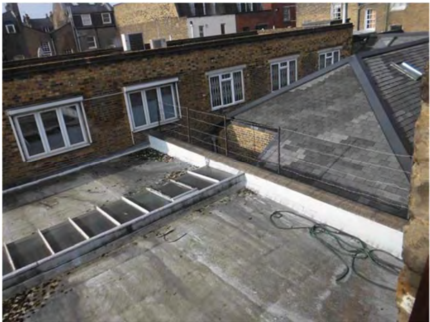
Photograph 8 - View from front building of lower roofs
