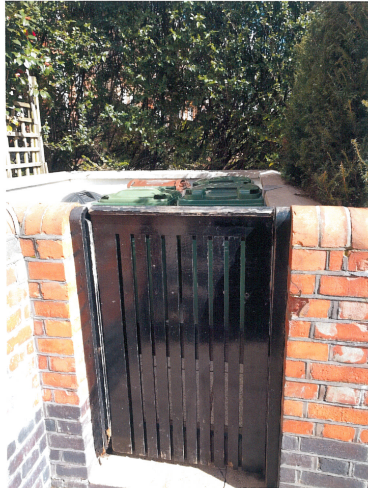
Door to Existing Bin Storage Area
