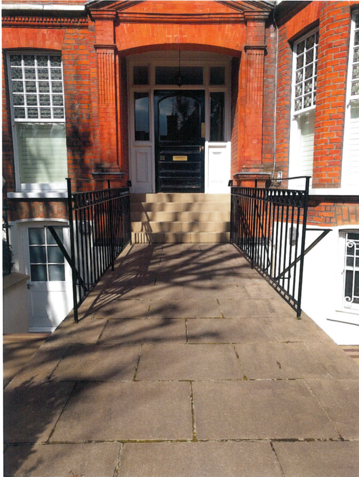
Existing Path and Front Door
